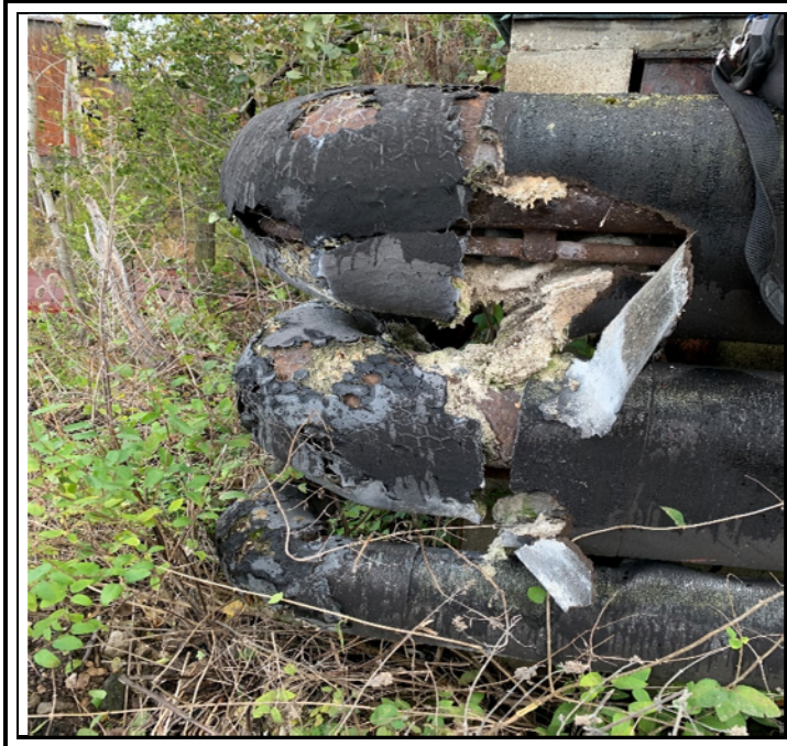
Photo 3 – Typical pipe insulation between Points B and C
