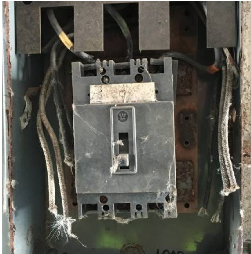
PACM cloth wrap on electrical wiring
